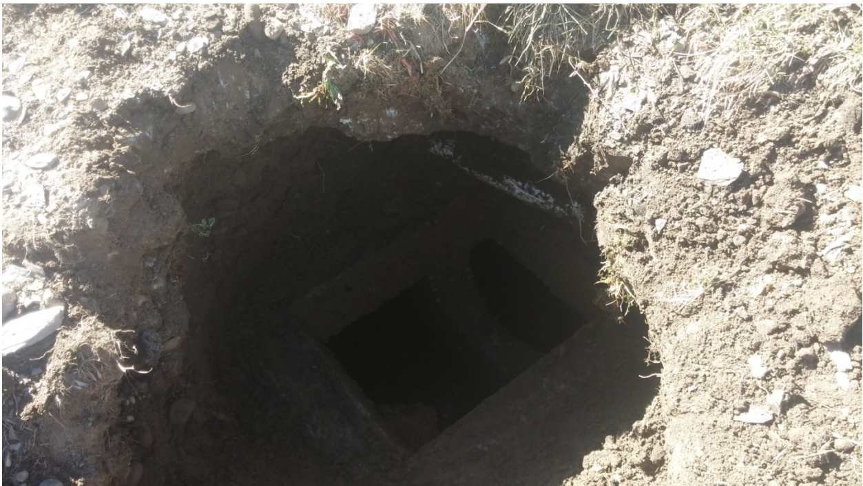
Photo 2 Camp Rising Sun ED Hall Septic Tank: March 6, 2016 Inlet opening cover removed.
