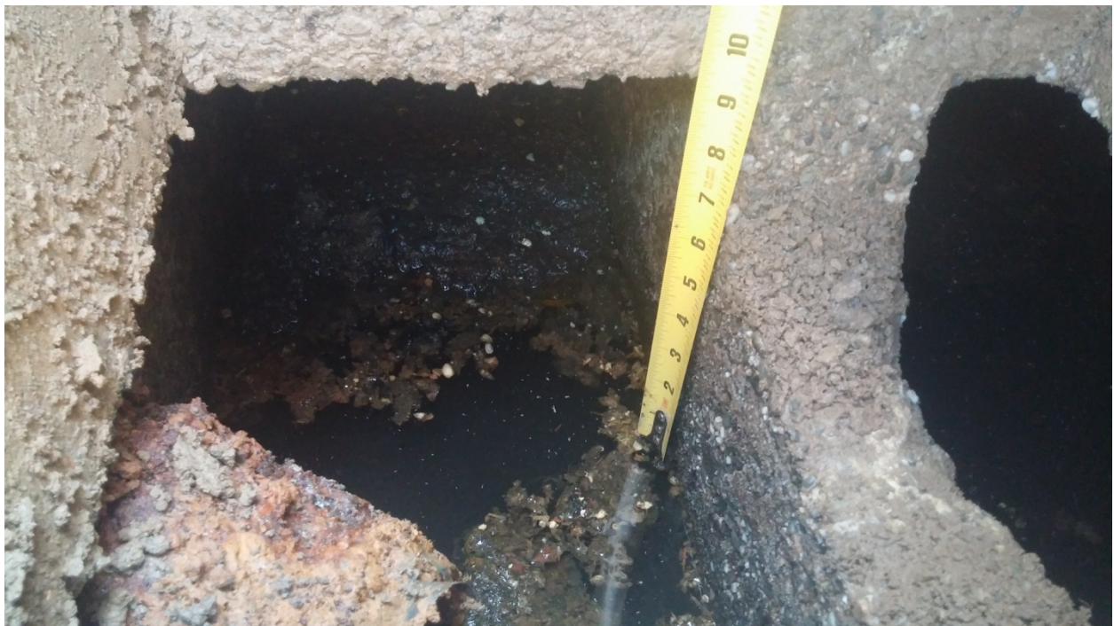
Photo 4 Camp Rising Sun ED Hall Septic Tank: March 6, 2016 The measurement shown indicates appropriate effluent height and air space.
