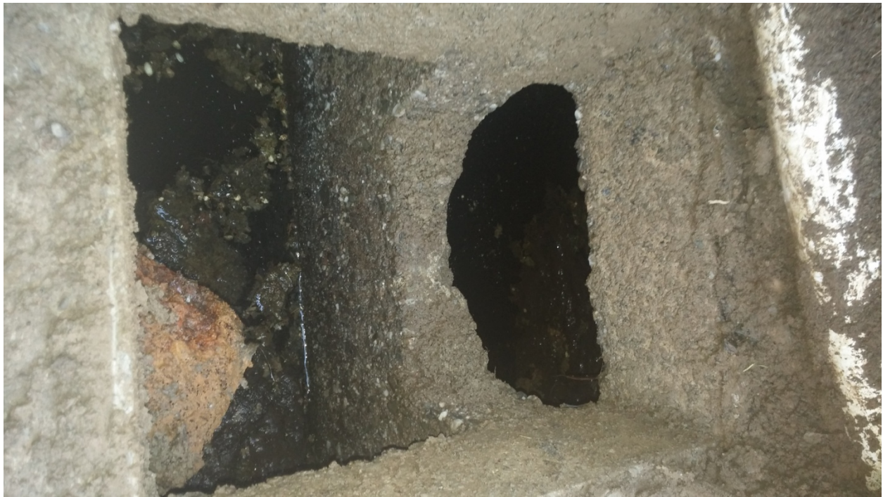
Photo 3 Camp Rising Sun ED Hall Septic Tank: March 6, 2016 Inlet opening with baffle shown provides sufficient access to service the septic tank in a legal and safe manner.
